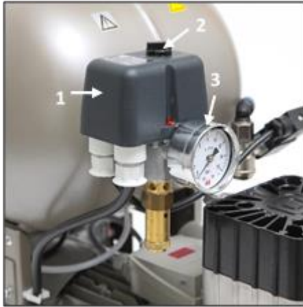
Fig. 5: Switching the compressor
