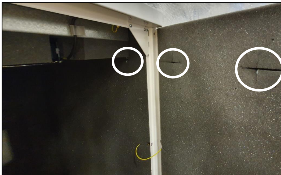
Fig. 16: Position of the clamps in the cabinet
