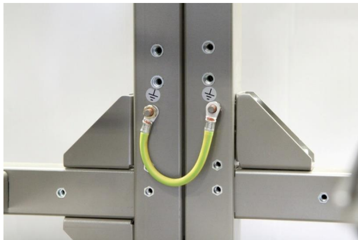
Fig. 8: Bonding the frames
