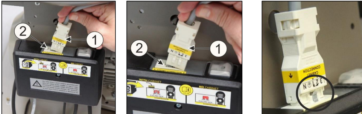
Fig. 11: Connecting a compressor installed in a cabinet
